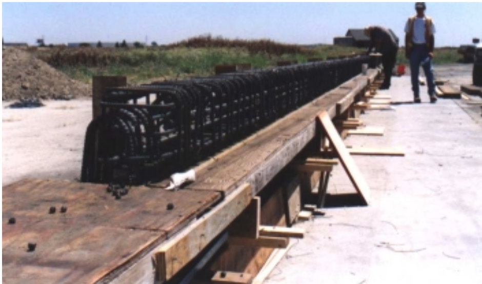
Figure 2-5 Steel Placement for Beam Section
