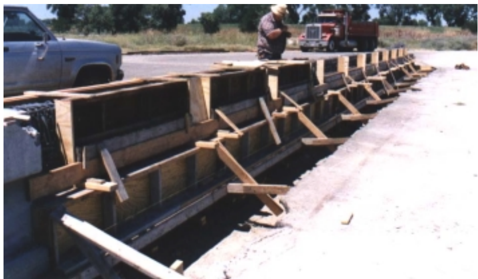
Figure 2-6 Form Placement for Beam Section
