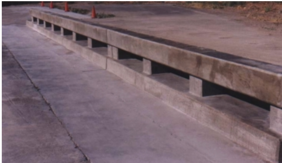
Figure 2-11 Completed Type 80 Bridge Rail
